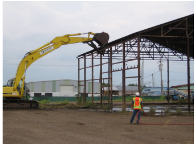
Dismantling of metal warehouse (storage building).
